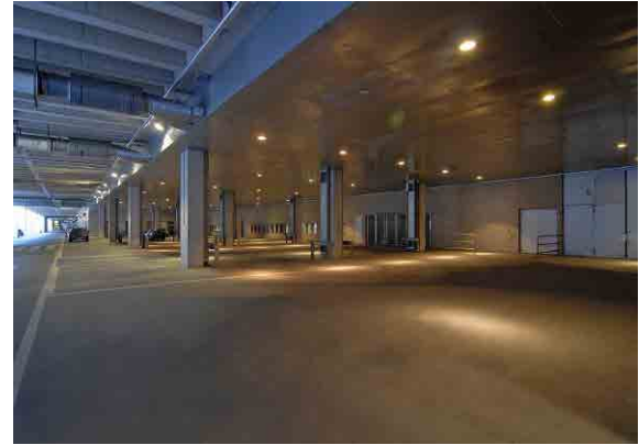
Car park level U1
